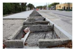
Image 17: The image above shows the construction of integrated planters with stormwater. The image to the right is the new recommended standard for tree pit design in NYC; integrating stormwater management, street trees and tree protection.
