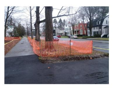
Image 3: This is an example of tree protection at a construction site. While the trees are protected and the disturbed roots were not torn, but cleanly cut; it could be argued that all disturbance to these trees could have been avoided if the site was accessed from the rear alley only.
