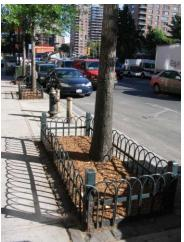
Image 16: Shows a comparison of how some sidewalk tree pits in Saratoga Springs are constructed, versus an example of how a tree pit is ideally constructed. The larger protected tree pit offers more rooting volume, access to moisture and oxygen for the tree, which will likely cause less damage to the sidewalk.
